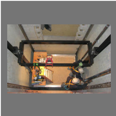
Lift Repair And Modernization
