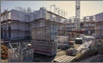
House Construction Service
