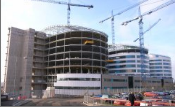
Hospital Construction Service
