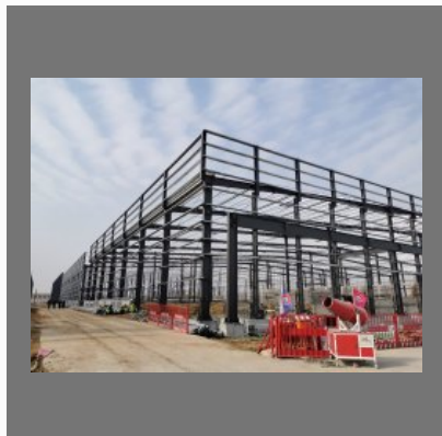
Prefabricated Steel Building Structure
