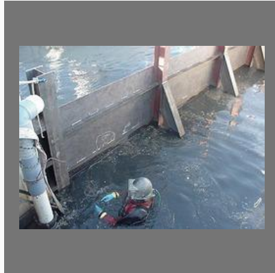
Underwater Cofferdam Installation Service
