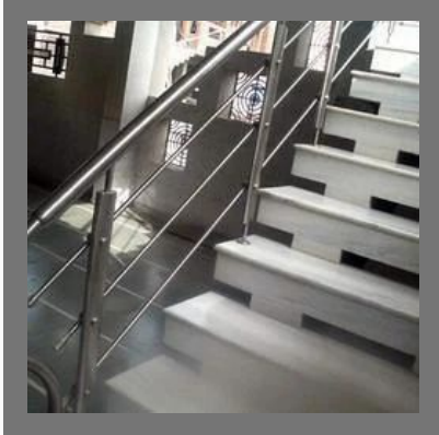
Stainless Steel Staircase Railing
