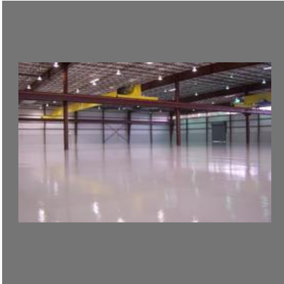
Industrial Epoxy Flooring
