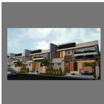
Residential Villa Construction
