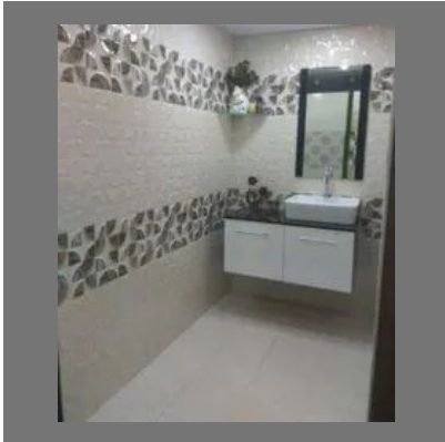
Toilet Civil Plumbing Service
