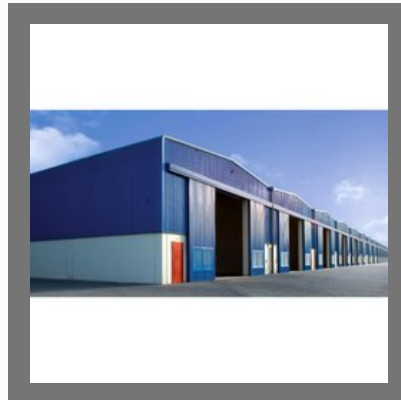
Prefabricated Industrial Structures
