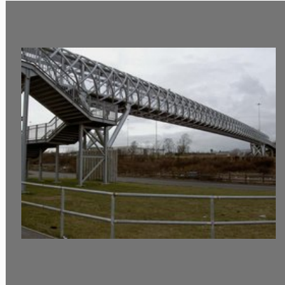
Self Make Metal Foot Over Bridge
