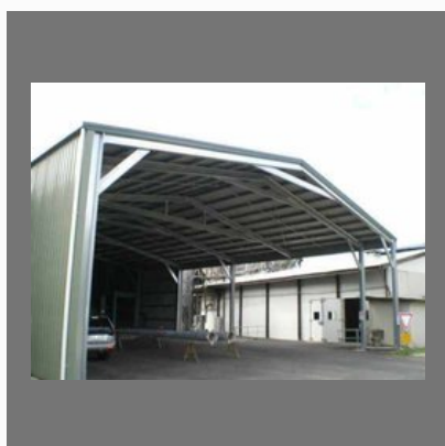
Prefabricated Factory Shed
