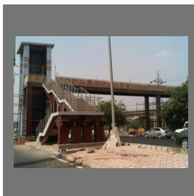
M.D. Foot Over Bridge
