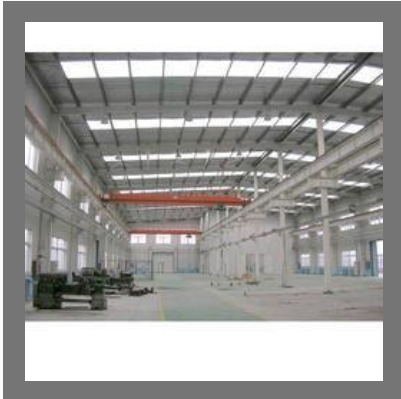
Truss Fabricated Structure
