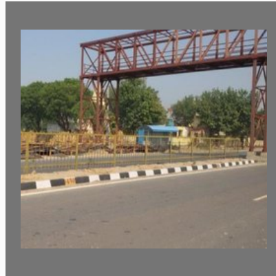
Bharat Udyog Foot Over Bridges
