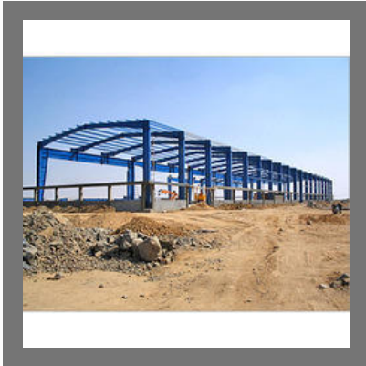
Industrial Pre Engineered Building
