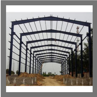
Pre Engineered Building
