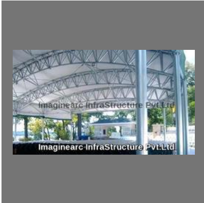
Space Frame Canopy
