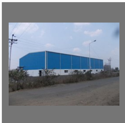
Stainless Steel Prefabricated Factory Shed
