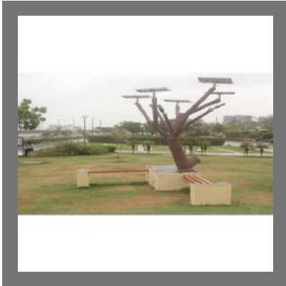
4.2 Kw Solar Power Tree
