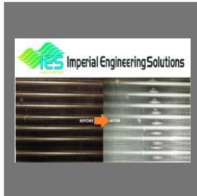
AHU Coil Cleaning Service
