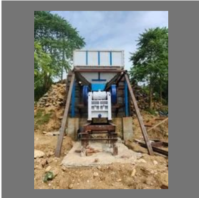
Automatic Stone Crusher Plant
