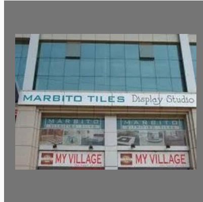
ACP signage work
