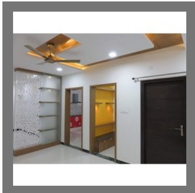
Living Room Gypsum False Ceiling
