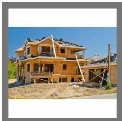
House Construction Services
