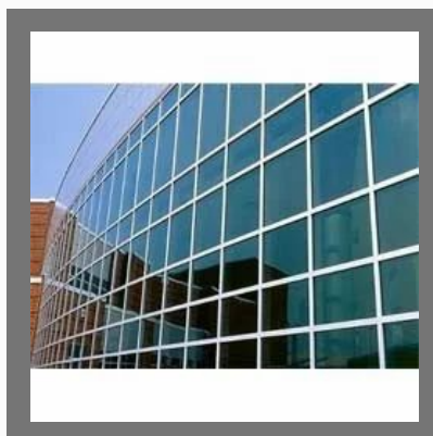
Structural Glazing Work
