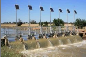
Working Group On Modernization Of Irrigation Systems
