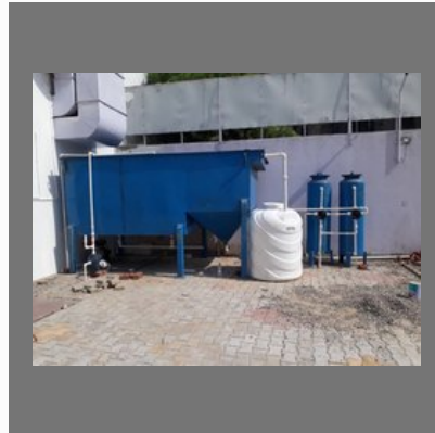
Sewage Treatment Plant
