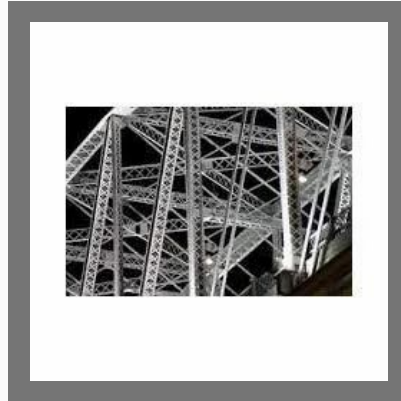
Angular Truss Fabrication
