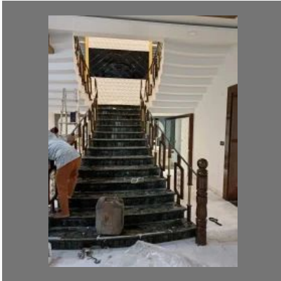
Designer Staircase Railing
