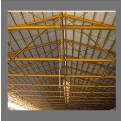
Angular Truss Fabrication
