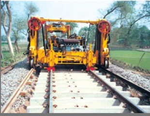
Railway Tracks Construction Service
