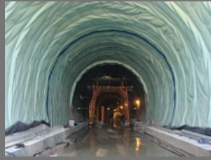
Railway Tunnels Construction Service
