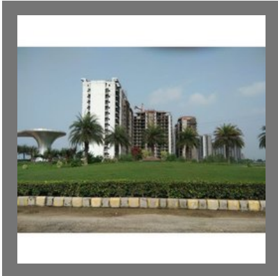
School Building Construction Service
