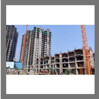
Flat Construction Service
