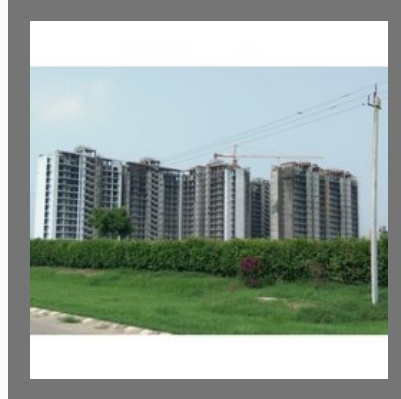
Apartment Construction Service
