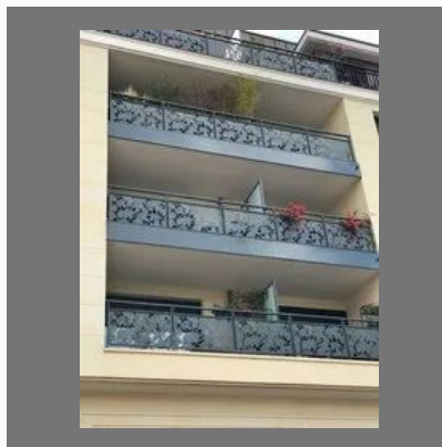
Stainless Steel Railing
