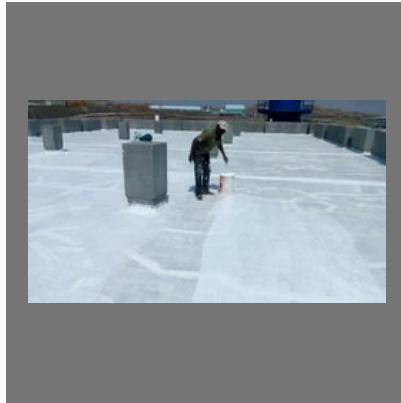
Water Proofing Treatment
