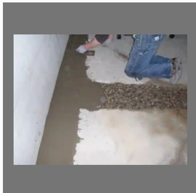
Basement Waterproofing Service
