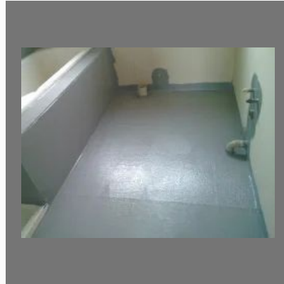
Bathroom Waterproofing Services
