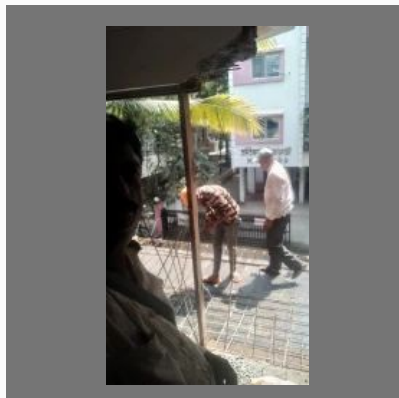
Civil Maintenance Works
