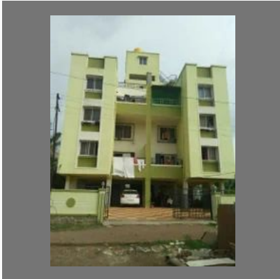
House Construction Service
