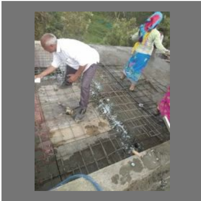
Civil Engineering Service
