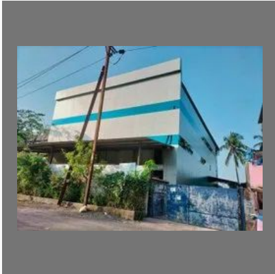
Glass Structural Glazing in Mumbai
