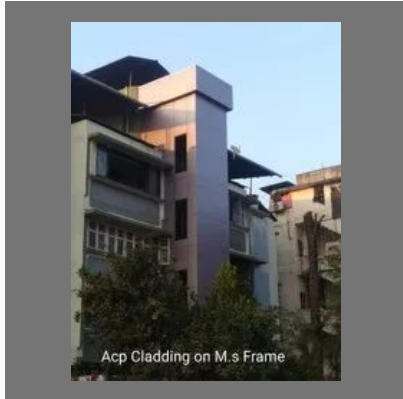
ACP Wall Cladding
