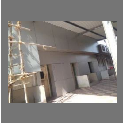
ACP Cladding Installation Service
