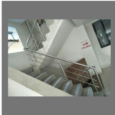
S S Railing
