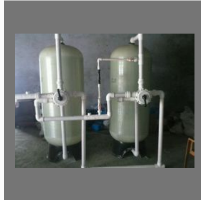
Industrial Water Softener
