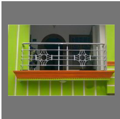
Stainless Steel Balcony Handrail
