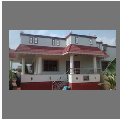
Kerala Balcony Railing
