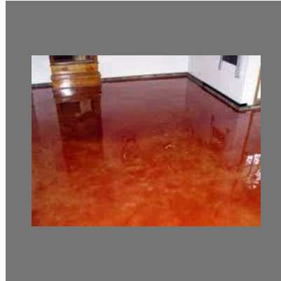
Epoxy Floor Paint
