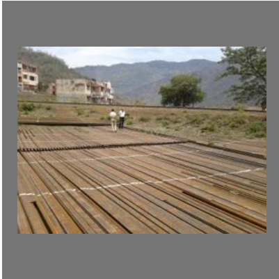
Narrow Gauge Rail Track
