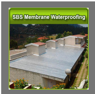
SBS Membrane Waterproofing
