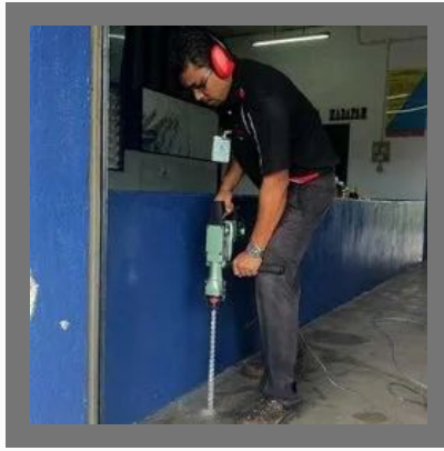
Drilling Termine Control Services
