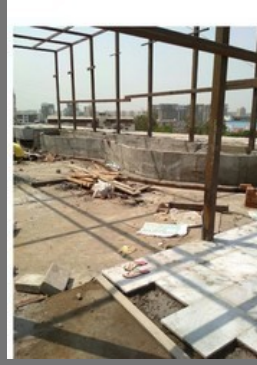
Tiles Fitting Services For Office
