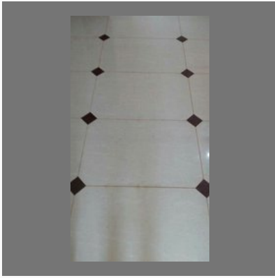
Tiles Fitting Work
