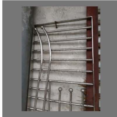
SS House Railing
