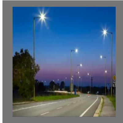
Led Street Lights.
