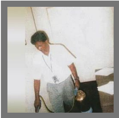
Post Construction Anti Termite
