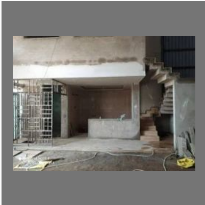
Guest House Construction
