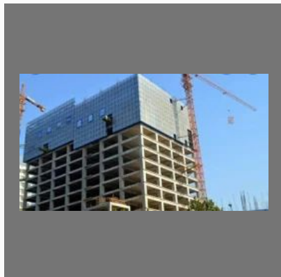
Commercial Mall Constructions
