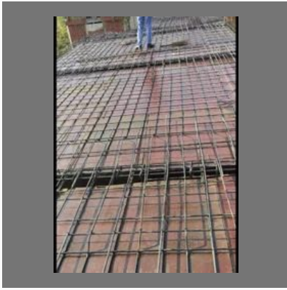
Warehouse Buildings Construction Services
