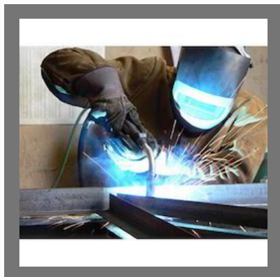
Mild Steel Fabrication Work
