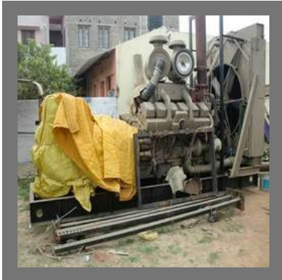
Generator Repair Service
