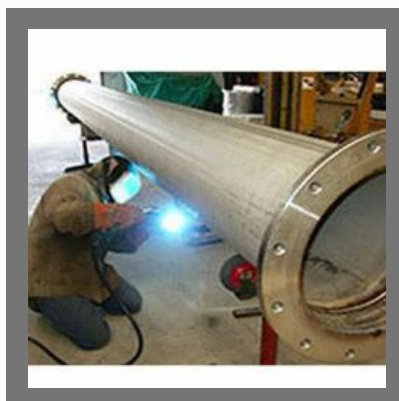
SS Pipeline Fabrication Services
