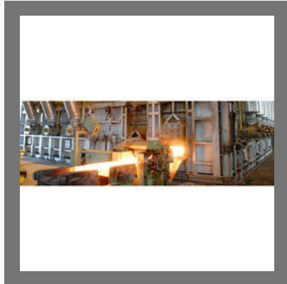
Re-Heating Furnacing Steel Rolling Mill Plant
