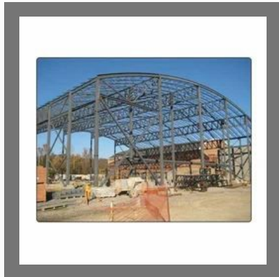
Iron Structural Fabrication Work
