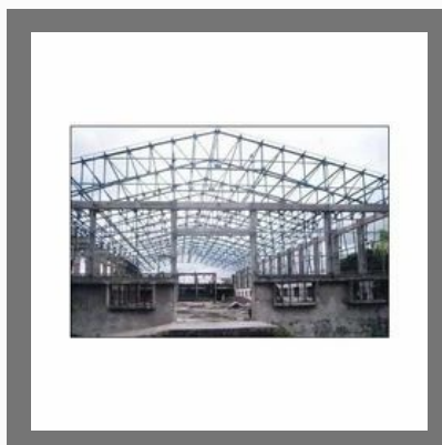
Heavy Structural Fabrication Work
