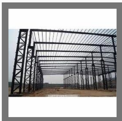
Heavy Structural Erection Service
