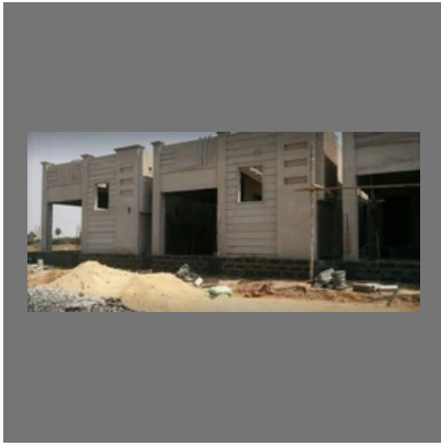
School Building Construction Services
