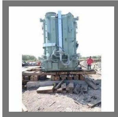
Transformer Loading, Unloading, Shifting Service
