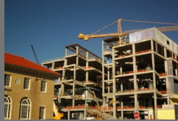
Building Construction Services
