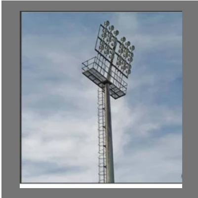
Stadium Lighting Pole
