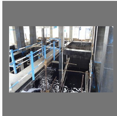
Concrete Protective Coating
