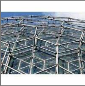
Steel Structures Service
