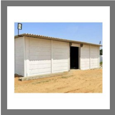
RCC Precast Labour Quarter
