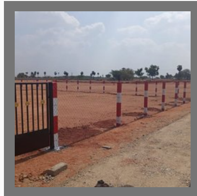
Wire Fencing Service
