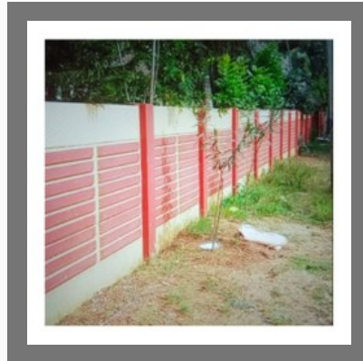
Concrete Precast Compound Wall
