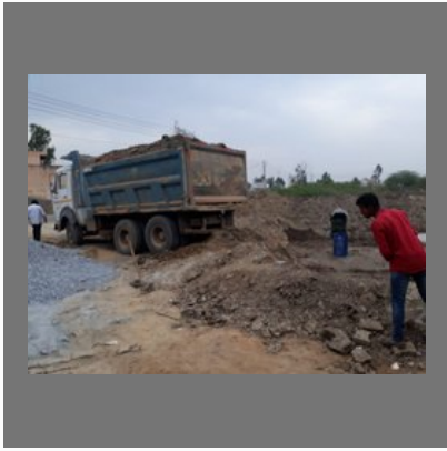
House Construction Works
