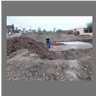
House Construction Works
