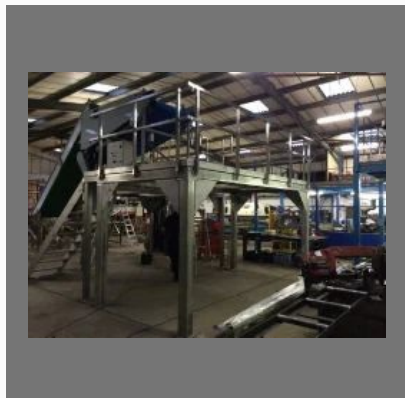
Heavy Industrial Structure Fabrication Work
